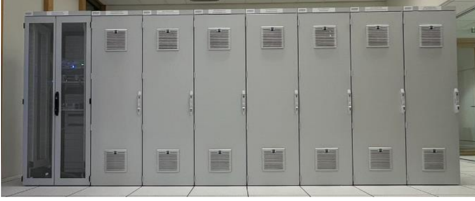
Figure 2 – View of the VSC-HVDC bipolar control replica in the real-time simulation lab
